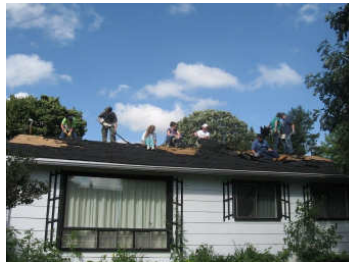
New roof for DW
