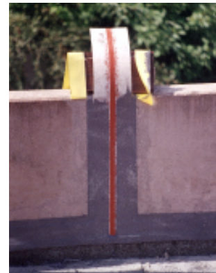
RedLINE 06 being installed
