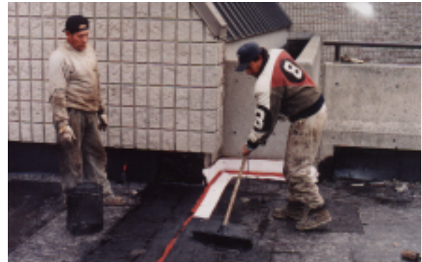
RedLINE 20 being installed
