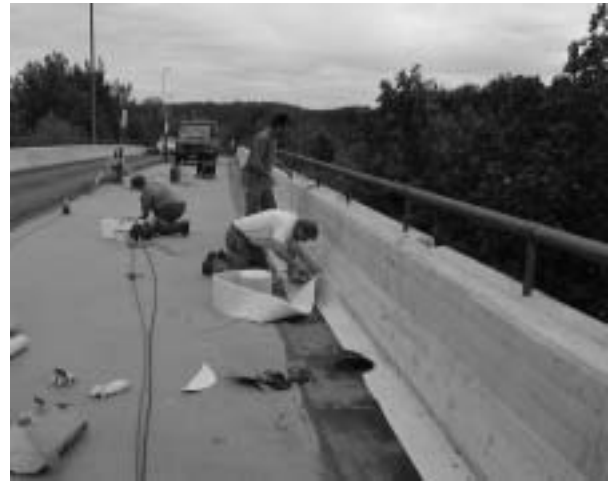
RedLINE Flashing being installed
