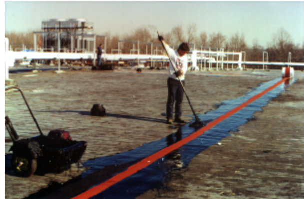
RedLINE 240 being installed
