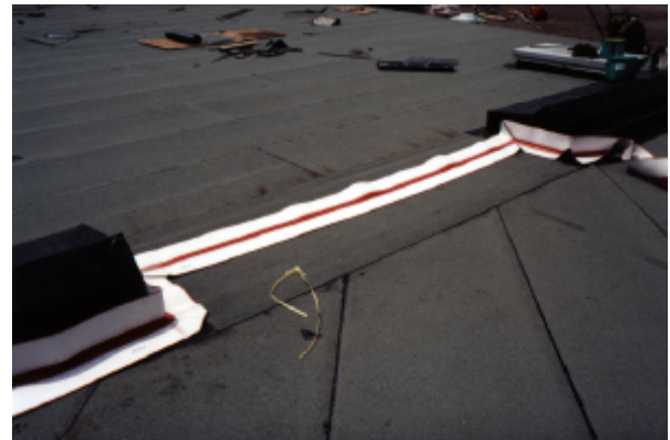
RedLINE 40 being installed
