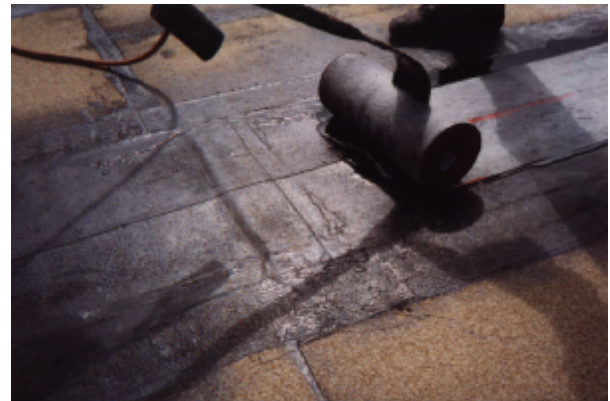
RedLINE 20G being installed
