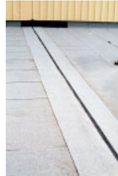
FlamLINE installed in a torch down system
