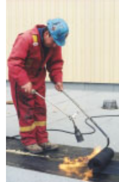
FlamLINE installed in a torch down system
